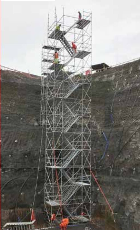
19 Torre escala industrial
